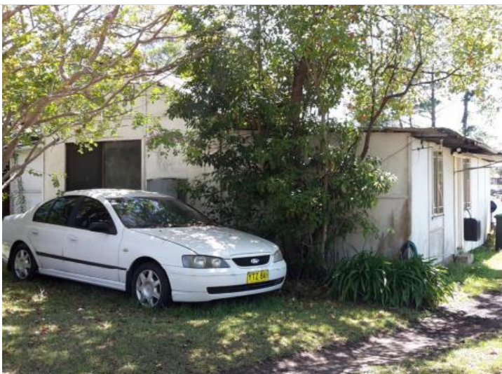
Photograph 15: Residence at No.3 Quarry Road. Structure generally constructed with fibre cement clad walls and corrugated fibre cement roof.
