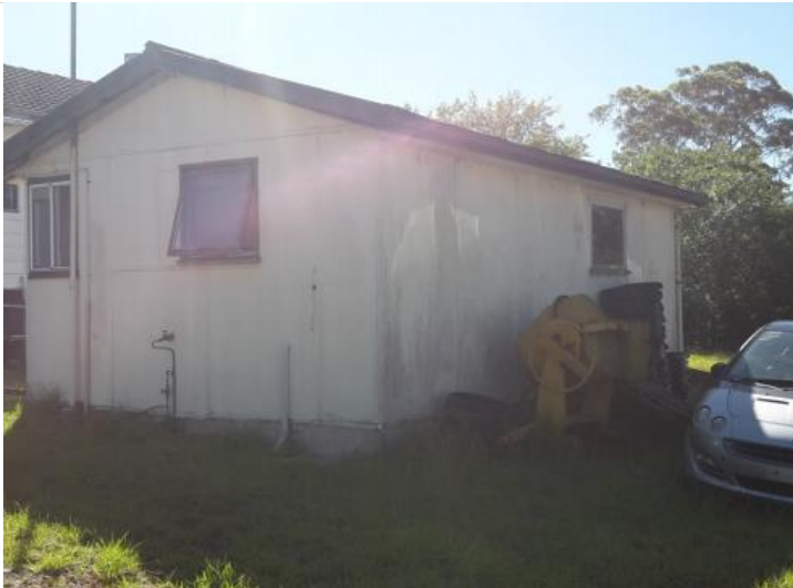
Photograph 14: Detached granny flat/garage, No.4 Vineys Road. Generally constructed with fibre cement clad walls and corrugated fibre cement sheet roof.
